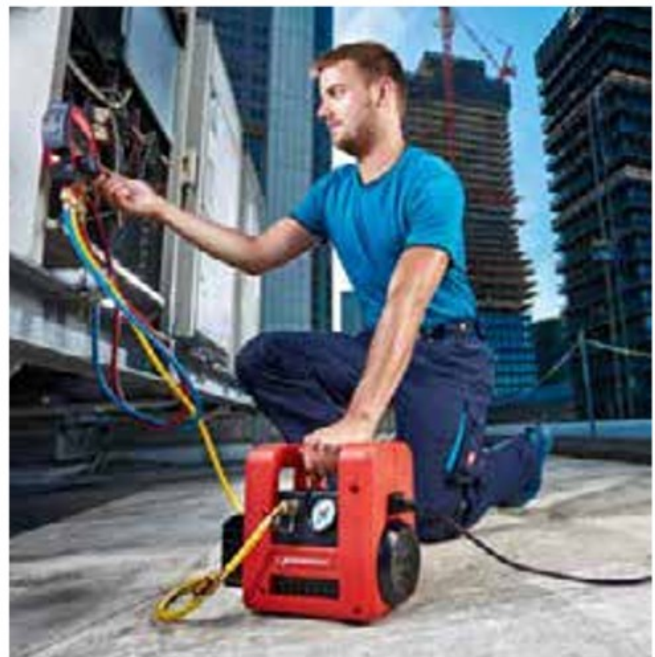
ROAIRVAC R32 1.5—vacuum pump in use with the digital manifold ROCOOL 600
